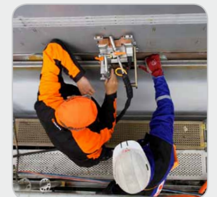
Operation is easy to instruct, plus all welding regulation is set from the carriage unit, reducing set-up time and making distance work easy.
